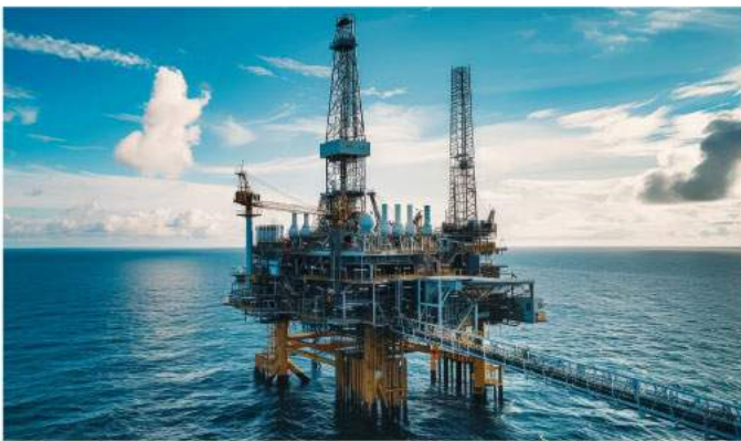
Onshore and Offshore Rigs
